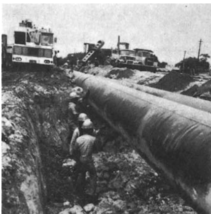
Hand cleaning. The 30-in. and 36-in. crude lines were cleaned by hand to expose corroded areas and prepare for tape-wrapping.
