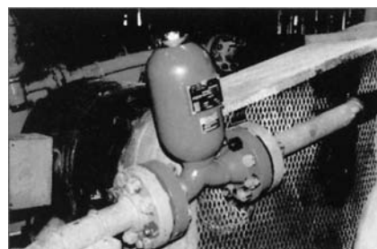
Figure 9. Flow-through pulsation dampener (Courtesy of Ormet Aluminum Mills Products Corporation, a Hannibal Rolling Mill Division).
