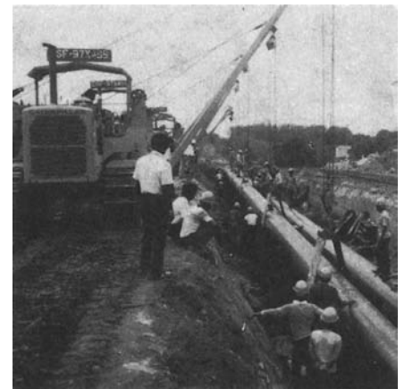
Gradual lowering. A full sweep of the total transition length is made by lowering each line 6 in. or less at a time. The procedure is repeated until the lines finally reach desired profile elevations.
