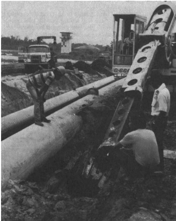
Excavation begins. Ten-foot soil plugs remained at 50-ft centers to act as temporary pipe supports for the 36-in. line.
