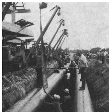
Lowering lines. The two lines, full of crude oil, are gradually lowered with the use of six sidebooms.
